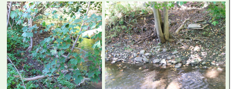
Fig. 10. The visual survey found signs of bank degradation such as "J-trees" indicating slope movement. In the channel, larger clasts lying on top of gravel-sized sediments are another indicator that sediment is being removed from the banks.
